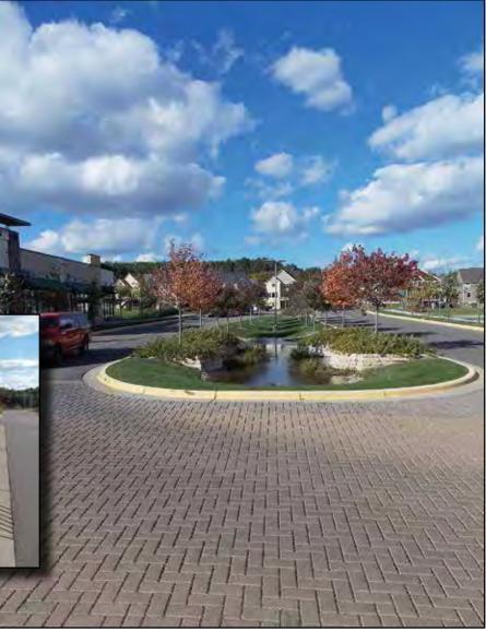
Median raingarden showing pervious pavers at intersection. Inset: Median raingarden showing curb cuts to direct runoff.
